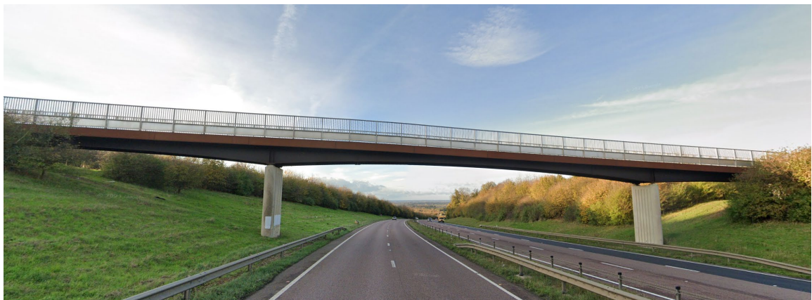
Plate 3.1 Example of a steel composite girder footbridge
