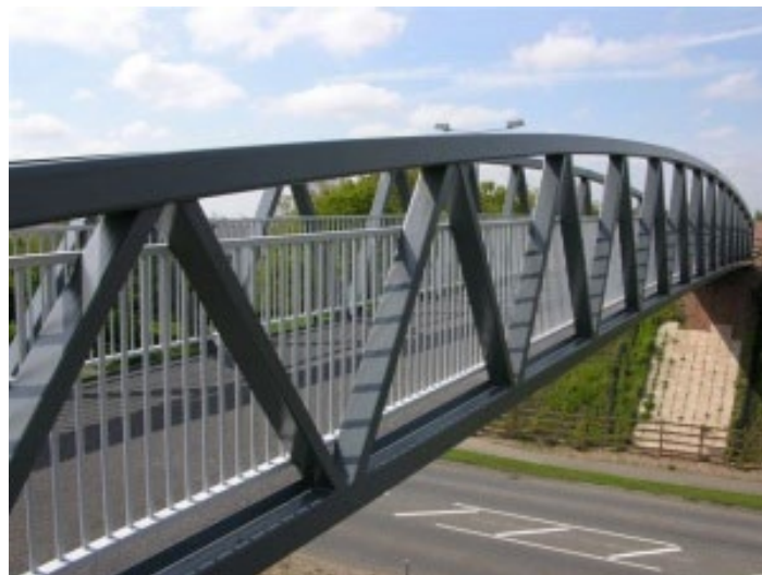
Plate 6.3 Example warren truss structure (3)
