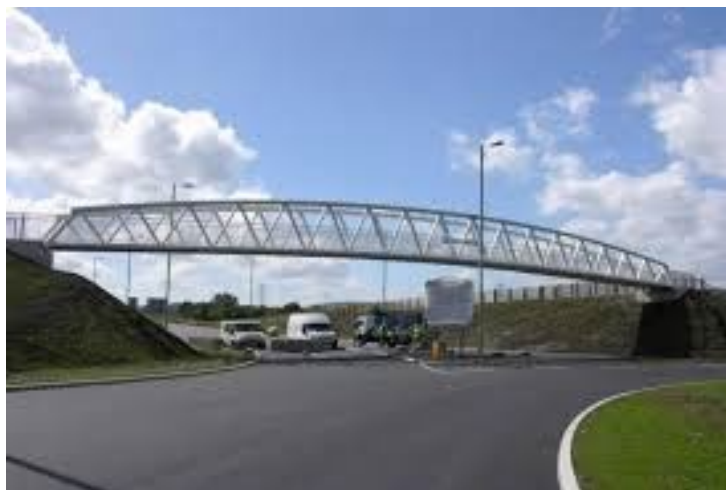
Plate 6.3 Example warren truss structure (3)
