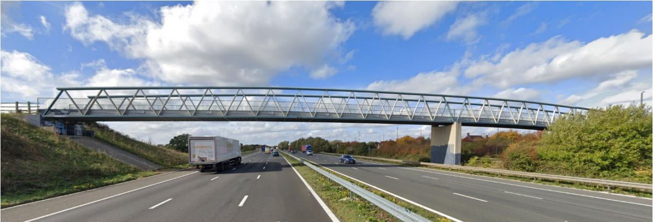
Plate 6.2 Example warren truss structure (2)
